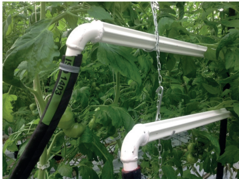
6: Heating elements of movable vegetation system (Walczak's pipe – primary diameter of 51 mm)
